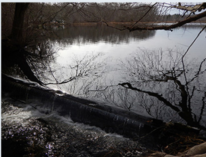
The fishway will be built at the Phillips Mill Pond Dam on the Nissequogue River. Photo credit: Vicky O'Neill/NYSDEC.
