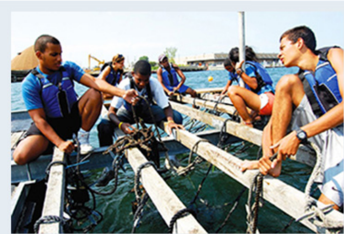
Students from Rocking the Boat help hang lines during the raft installation of the bioextraction project at the mouth of the Bronx River. Photo credit: Mark Dixon/ NOAA Milford Lab.
